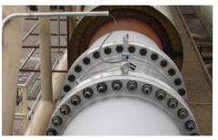
Flow measurement of heated water with the OPTISONIC 3400
