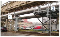
Supply line with flow straightener (1) and flowmeter (2)
