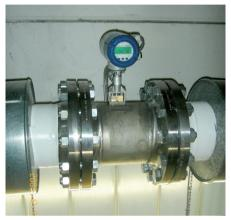
OPTISWIRL 4070 C with integrated pressure and temperature compensation (pressure loop is located on the back of the unit)
