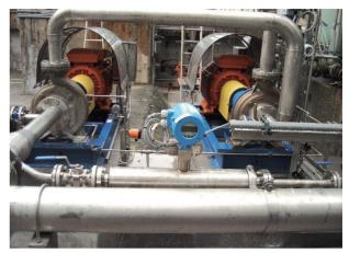
OPTIMASS mass flowmeters performing density measurement
