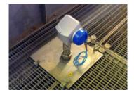
OPTIWAVE 6300 C mounted on top of hopper.
