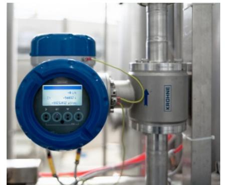
OPTIFLUX 6300 electromagnetic flowmeter
