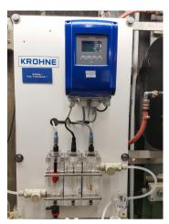
OPTISYS CL 1100 for pH- and temperature-compensated chlorine measurement
