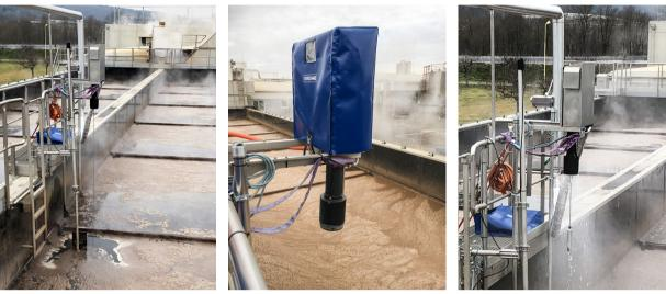
Measuring the sludge level in the clarifier
