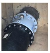
Infeed water measurement with the OPTIFLUX 2300 W
