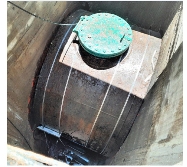
OPTISONIC 6300 mounted on DN2300 carbon steel pipeline
