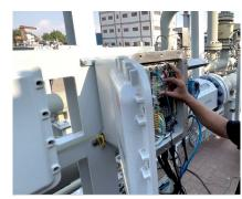
Connecting the remote converter of the ALTOSONIC 5 with a pressure transmitter
