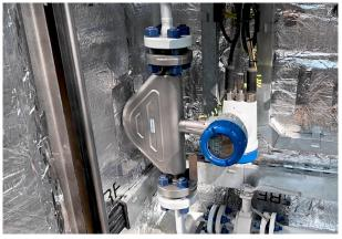
OPTIMASS 6400 Coriolis mass flowmeter mounted on the sampling system
