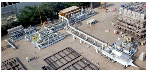
$Custody\ transfer\ metering\ system\ for\ crude\ oil\ with\ mobile\ prover\ and\ automatic\ sampling\ system$
