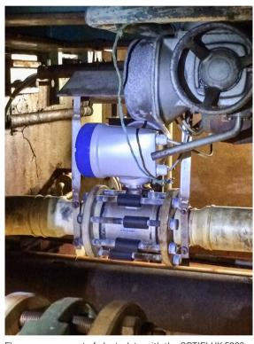
Flow measurement of electrolyte with the OPTIFLUX 5300 electromagnetic flowmeter
