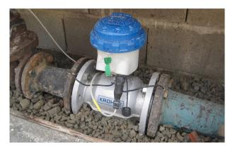
Measuring tube supported by gravel bed
