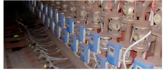
Automated monitoring of coolant leakage in a blast layer
