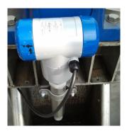
Installation of OPTIWAVE 5200 C with horizontal housing position
