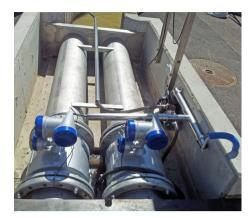
Installation of TIDALFLUX 2300 in sewage channel
