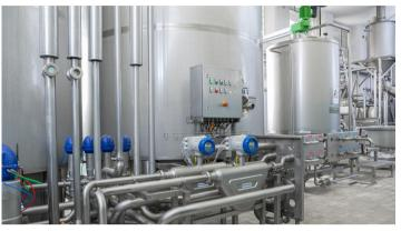
Installation of the OPTIMASS 6400 in front of the buffer tank
