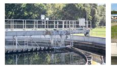
OPTISYS SLM 2100 and Radioline on the scraper bridge
