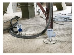
Level measurement in raw feed and grain silos
