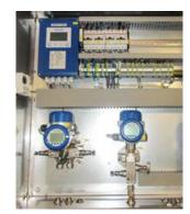
Control cabinet with KROHNE DP and pressure transmitters, temperature transmitter and flow computer
