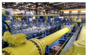
Core element of the fuel system are the two calibrated 16" metering sections (600 lbs) for a natural gas flowrate
