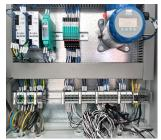
Remote converter of an OPTIFLEX 2200 level transmitter installed in a distributed I/O unit
