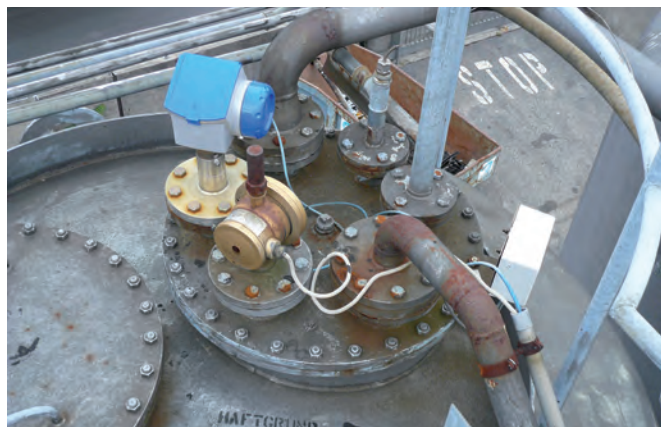
Installation on top of tanks
