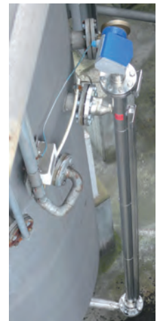
Bypass measurement on a 2-chamber tank
