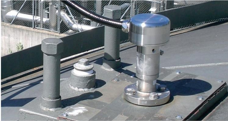
OPTIFLEX 1300: remote version of the probe assembly installed on a tank
