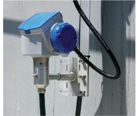
Remote version of the signal converter at eye level
