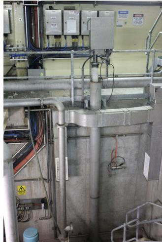
OPTISYS SLM 2100 mounted on a hopper of a primary sedimentation tank
