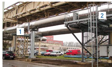
Supply line with flow straightener (1) and flowmeter (2)
