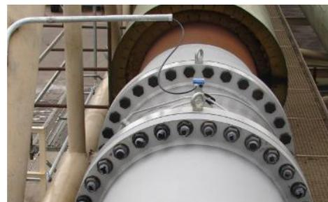
Flow measurement of heated water with the OPTISONIC 3400
