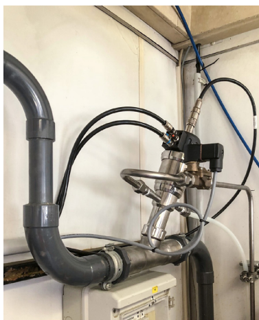
pH measurement with the SMARTPAT PH 8320
