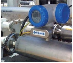
The OPTIMASS 7300 C with integrated concentration measurement
