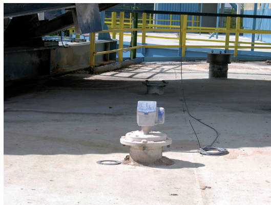
OPTIWAVE on the cement silo
