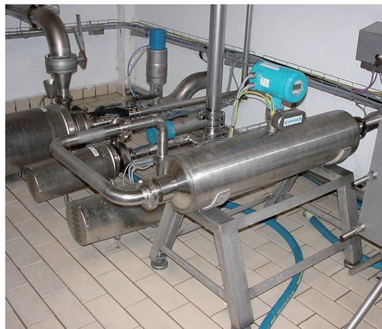
Mass flow measurements in pipeline for salt brine
