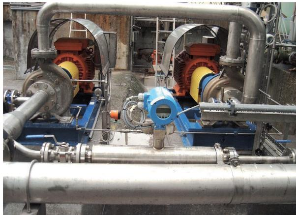
OPTIMASS mass flowmeters performing density measurement
