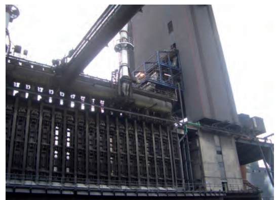
Coke oven battery with loading platform (top right)
