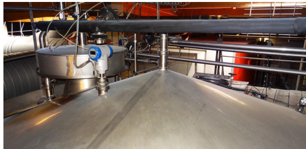
OPTIWAVE 5200 level transmitter on purified water tank
