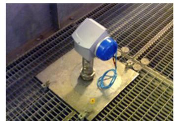
OPTIWAVE 6300 C mounted on top of hopper.
