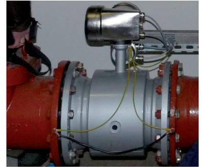
TIDALFLUX 2300 F in the discharge to the mixed water drainage system
