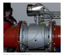
TIDALFLUX 2300 F in the discharge to the mixed water drainage system
