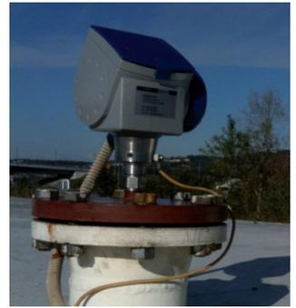
The OPTIFLEX 1300 C measuring on top of the separator
