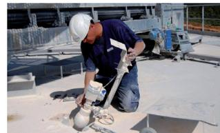
OPTIWAVE 6300 C [DN 150 (6")] measuring level in concrete silos
