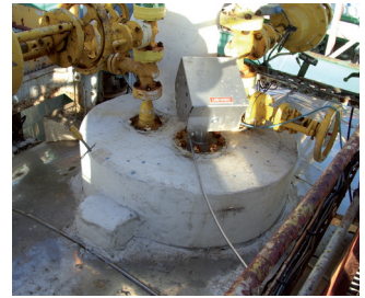
The OPTIWAVE 7300 C measures the chlorine level without contact
