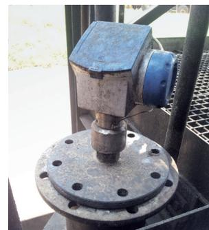
OPTIFLEX 1300 C mounted with nylon flange
