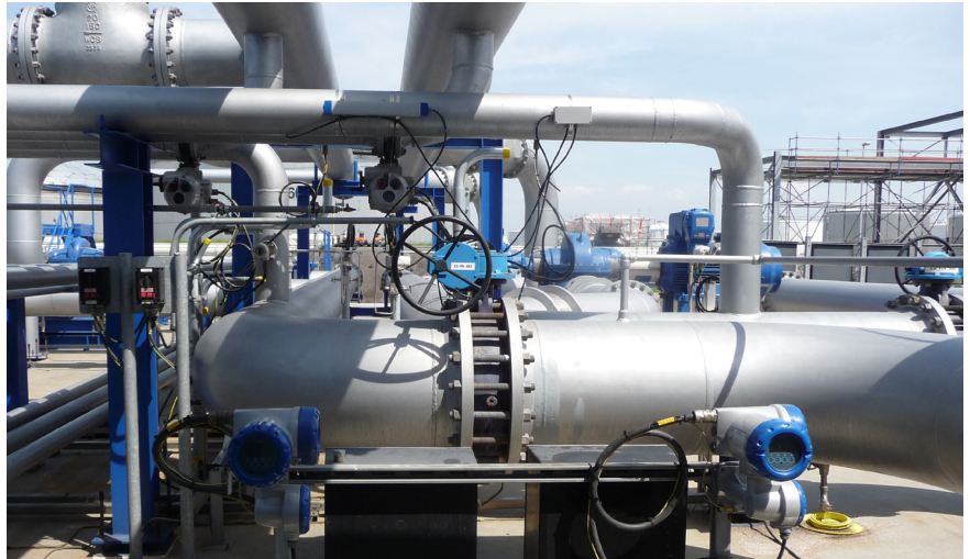
OPTISONIC 6300 with connection box and field housing
