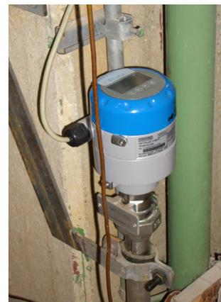
OPTIFLEX 1100 with reduced process connection
