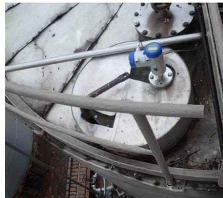
OPTIWAVE 5200 Ex d ia mounted on tank nozzle
