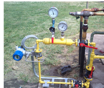
Installation of flowmeter with sandwich connection
