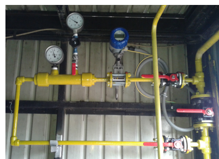
Vortex flowmeter mounted in a bypass line
