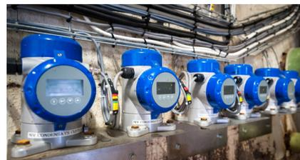
OPTIFLEX 2200 guided radar (TDR) level transmitters
