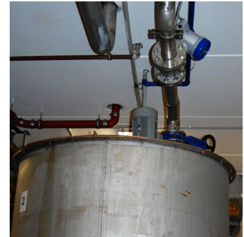
Installation of OPTIFLUX 7300 C for billing purposes
