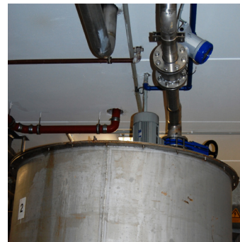
Installation of OPTIFLUX 7300 C for billing purposes
