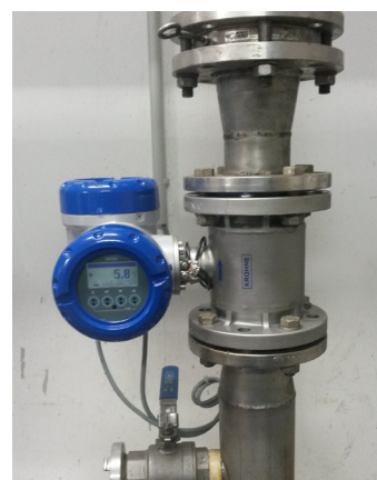
Flow measurement of fat for pump control
