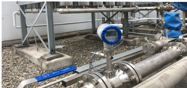
OPTISWIRL 4200 with integrated pressure and temperature compensation
