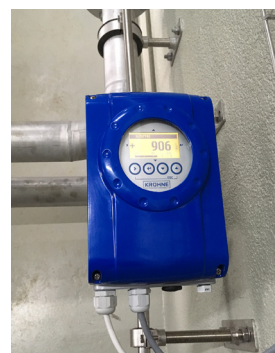
Flocculant measurement with the OPTIFLUX 1050
