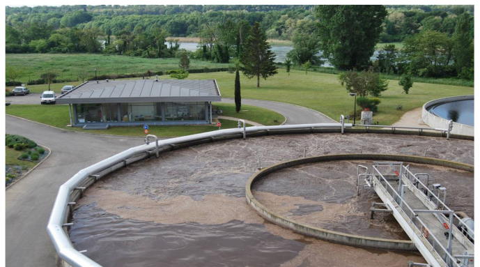
Wastewater treatment plant
