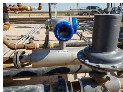
Crude oil measurement with the OPTIMASS 1400
